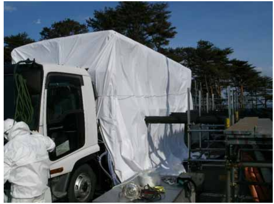
Installation of the cover
