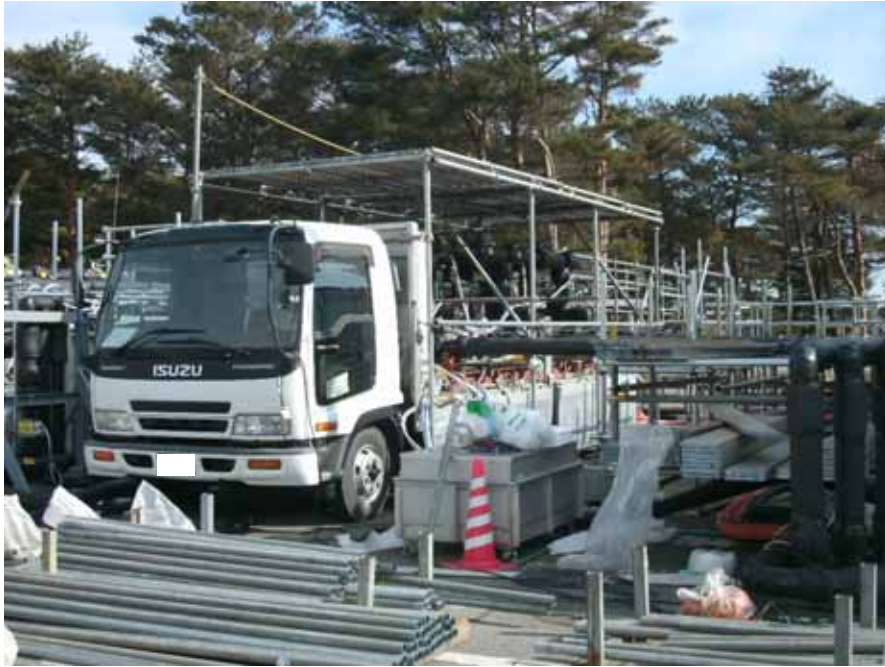
Installation of the frames
