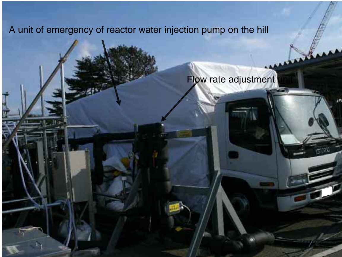
the Cover (emergency of reactor water injection pump on the hill)
