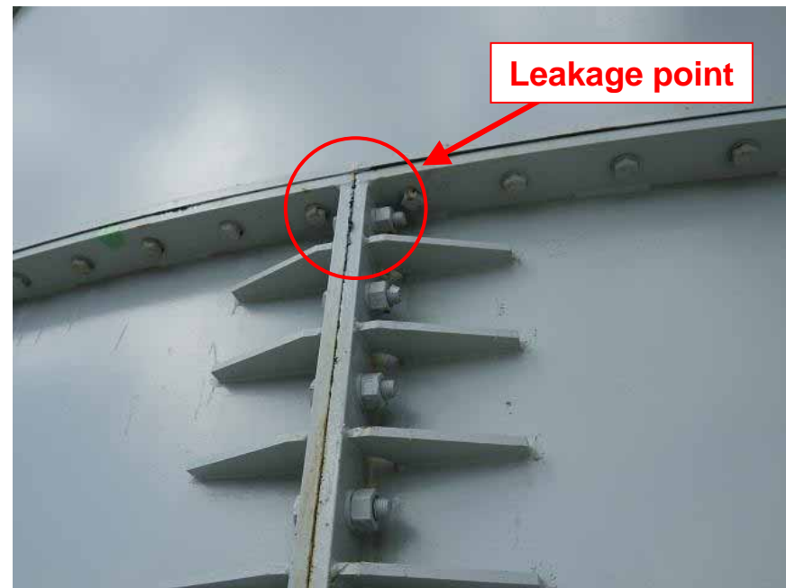
< Leakage point >
