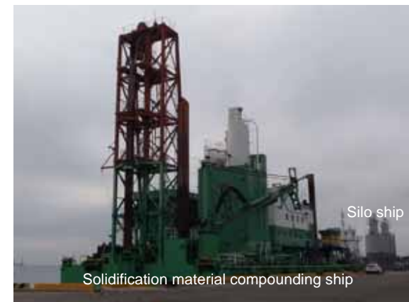
Picture 1 Work ships ( taken at Onahama Port )
