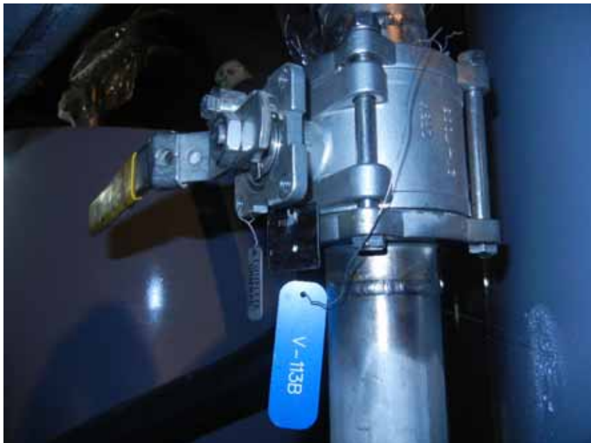
After removal of cover
