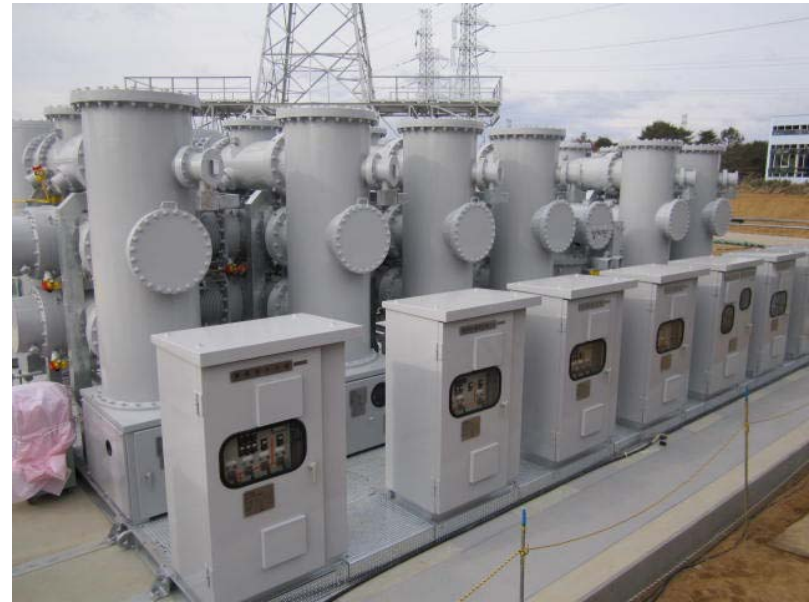
66kV switching facility (GIS)
