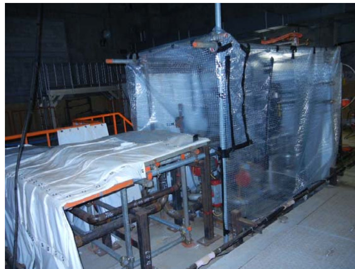
Situation of sheet curing
