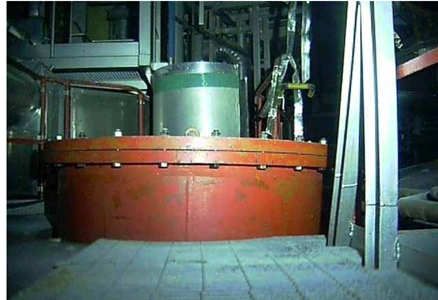
[Torus room southeast S/C manhole]
