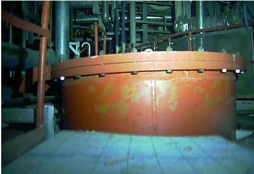
[Torus room north S/C manhole]
