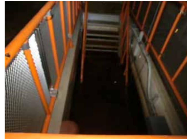
Unit 2 stair case (Northwest)
