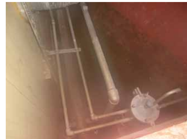
Unit 2 torus room (Northwest entrance)
