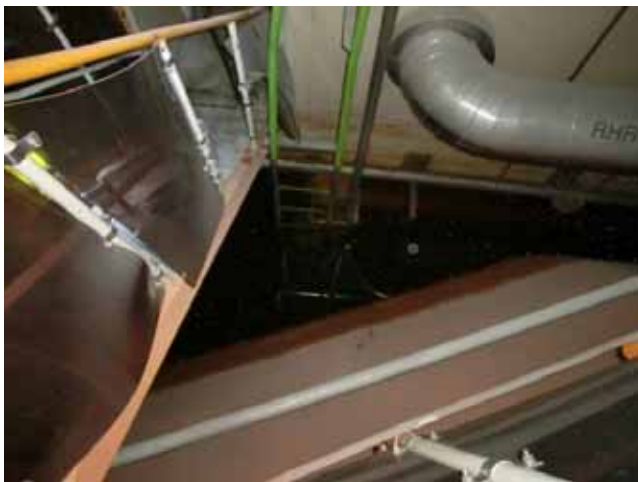
Unit 3 torus room (Northwest entrance)
