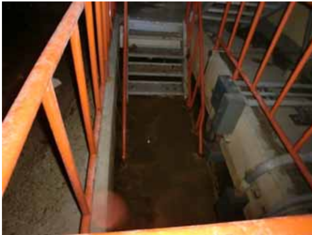
Unit 3 stair case (Northwest)
