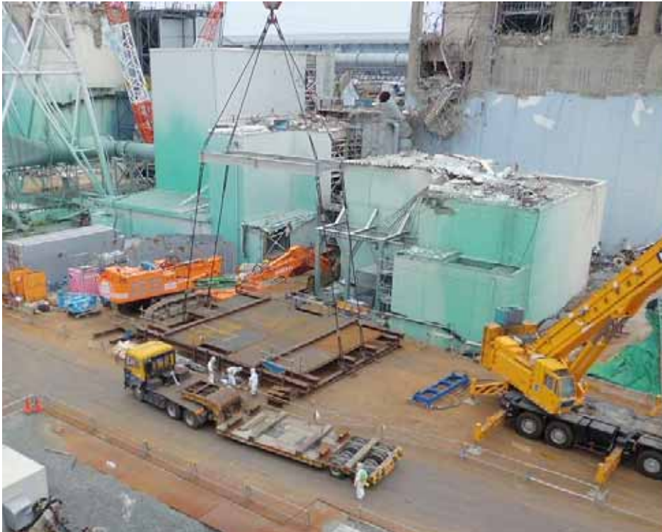
Before lifting up the protection platform
