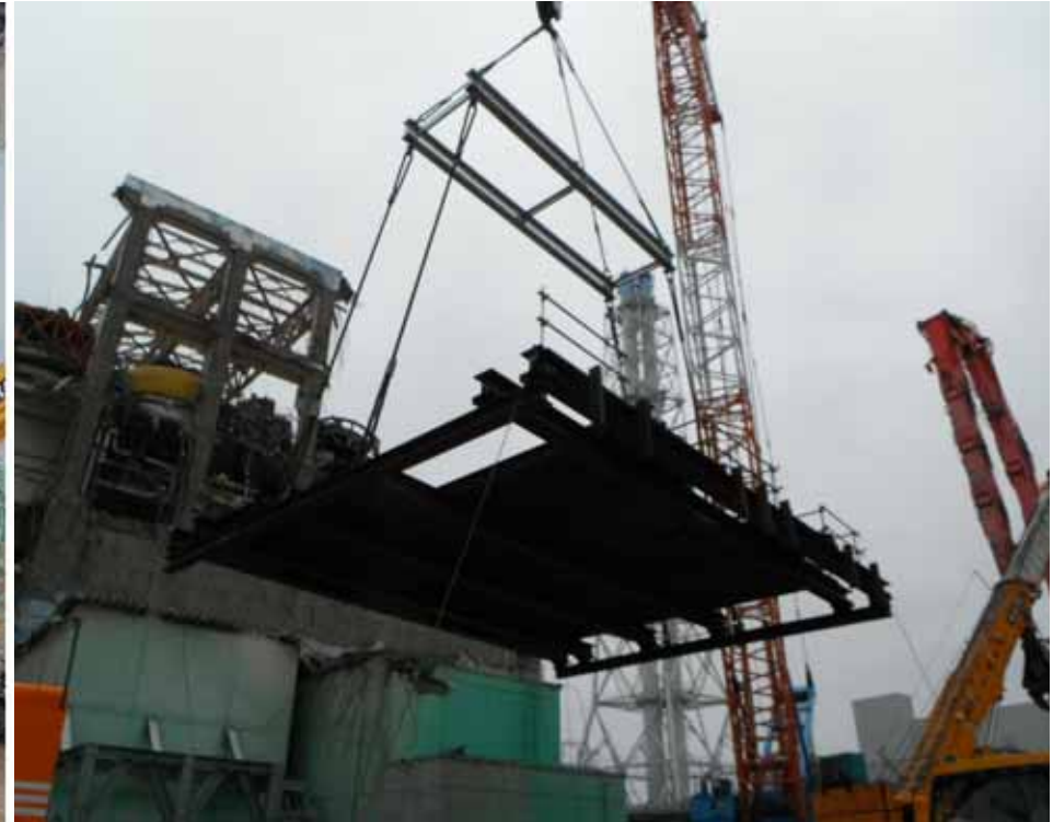
Lifting up the protection platform-1
