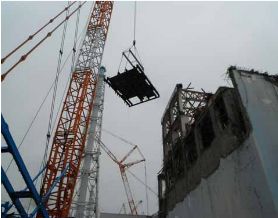
Lifting up the protection platform-2
