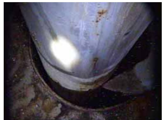
3. Penetration area on the floor
