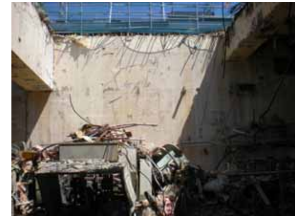
⑩ Wall on the SFP side (West)
