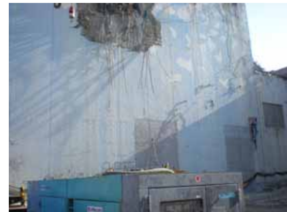
⑥ South wall (Exterior wall)
