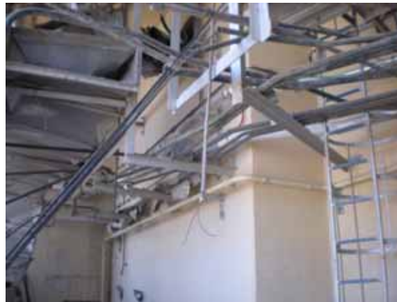
⑨ Wall on the SFP side (East)
