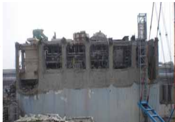
⑤ West wall (Exterior wall)
