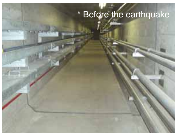
2. Inside of the duct
