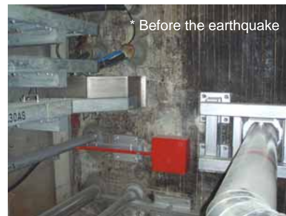
3. Inside of the connecting pit
