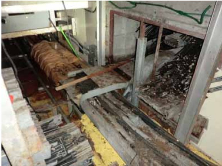
Before the water stop work (Photo taken on June 11, 2012)
