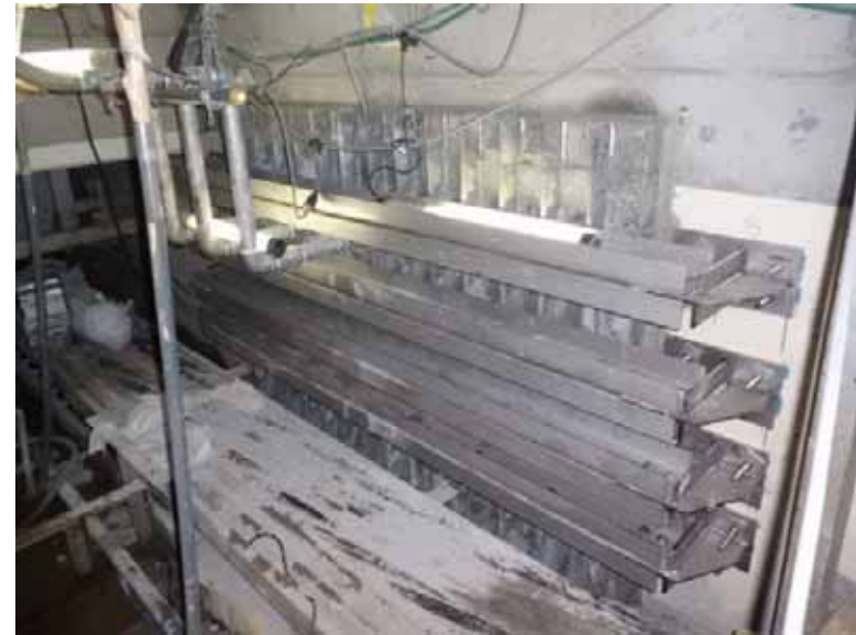
After the water stop work was completed (Photo taken on December 4, 2012)
