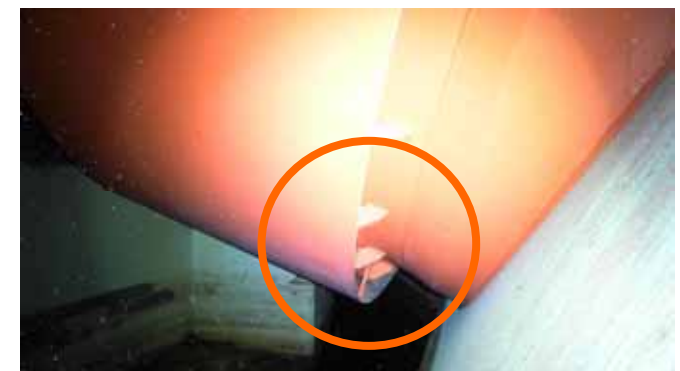
Lower part of vent pipe bellows cover
