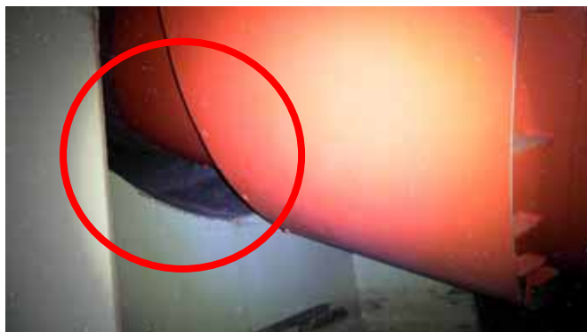
Edge of vent pipe sleeve
