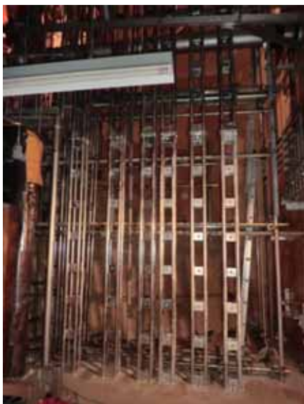
Figure 6 Steel posts installed condition
