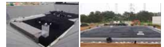
Underground water storage tank installation
