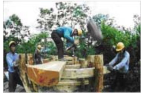
<Works to reconstruct damaged wooden path>
