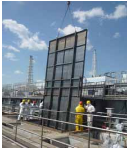
Steel plates were already installed (Unit 2) (completed by April 15)
