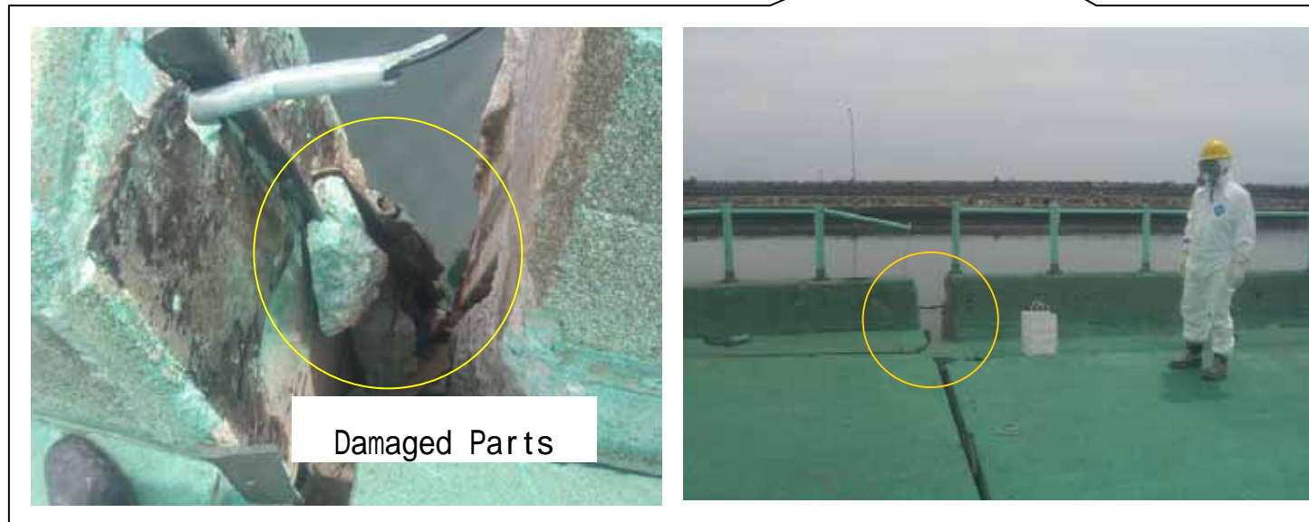
Shore protection Survey Result
