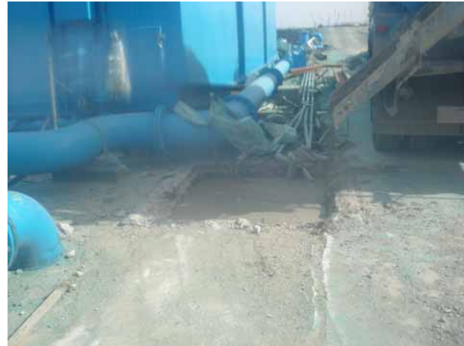
Concrete placement case [No.84]
