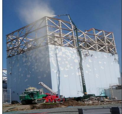
Dispersion of inhibitors by bending spray tower vehicle
