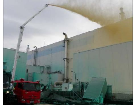
Dispersion of inhibitors by bending spray tower vehicle
