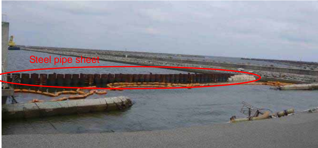
Status of steel pipe sheet pile
