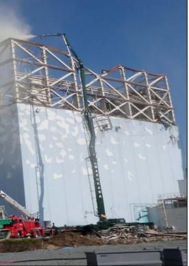
nhibitors by bending spray tower vehicle
