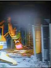
debris using Brokk emote control)
