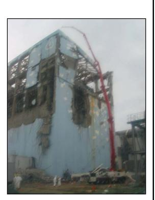
Dust sampling by the concrete pumping truck (May 23) Upper part of R/B, Unit 4
