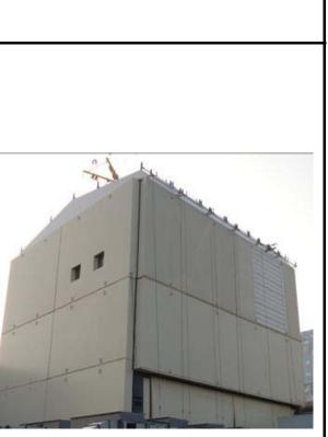
Completion of installation of roof panel on Oct. 14
