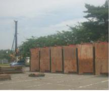
Shielding equipment to reduce exposure dose during outdoor work
