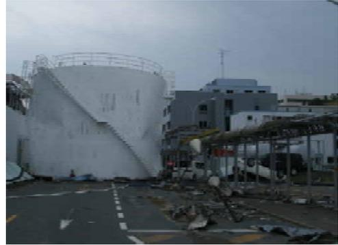
Fuel oil tank swept away by the tsunami and blocking a road
