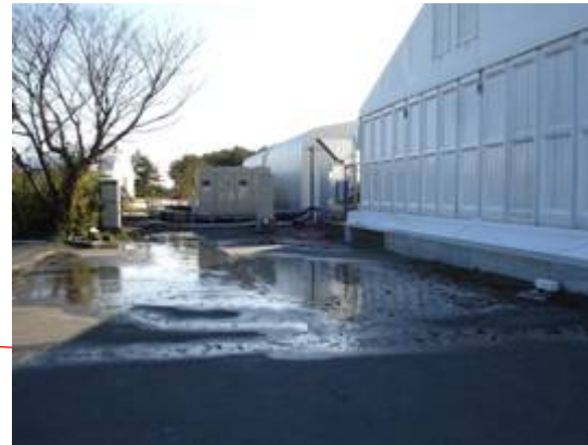
Status of leakage (puddles)
