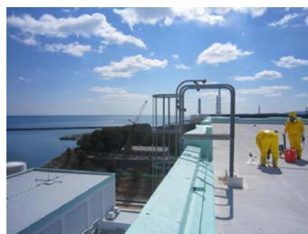
Work conditions on the roof
