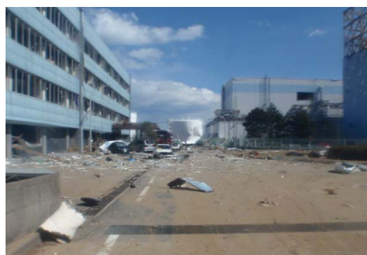
Former main office building with shattered windows (Unit 1 on the extreme right)
