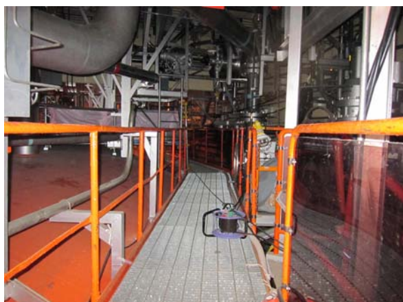
Condition of torus room (Unit 5, lighted)
