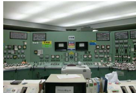
Restored lighting in main control room (Unit 4)
