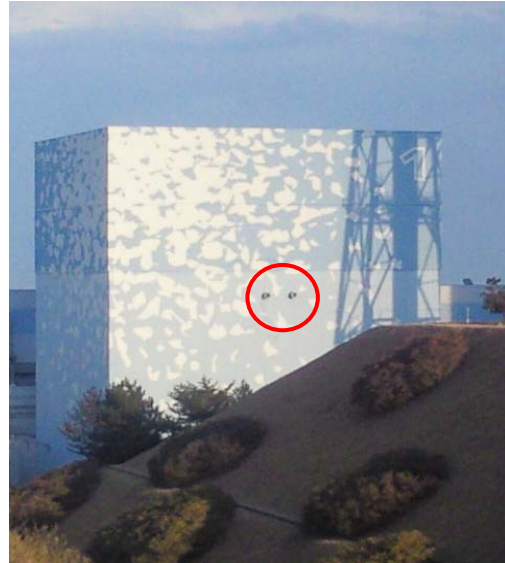
IC vent tube (commonly called as "Buta-no-hana")
