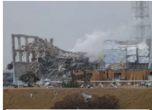
Damage to Unit 4 (right side in photo) (Unit 3 is on left side in photo)
