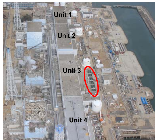
Condenser reversing valve pit of Unit 3
