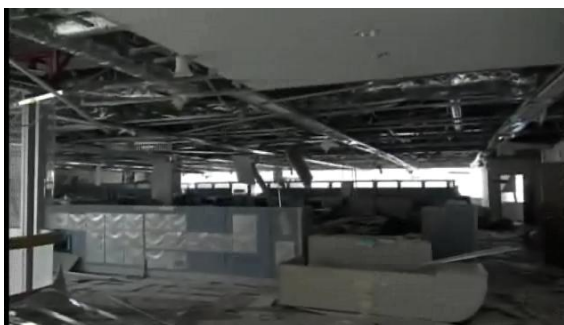
Main Office Building
