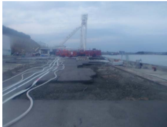
The fire-engine-based water injection from the Shallow Draft Quay
