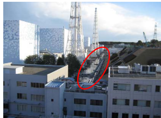
Entire areas of Units 1 to 4 flooded in the tsunami
