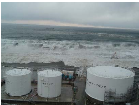
Tsunami destroying the breakwater over 10m tall and flooding over
