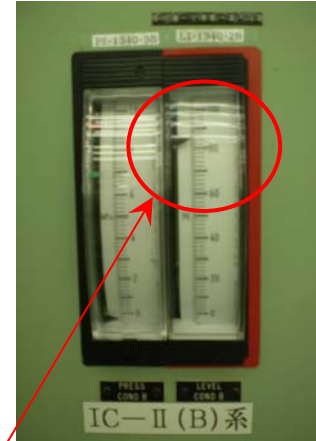
IC (B) steam pressure gauge and water level indicator (Photo taken later)
