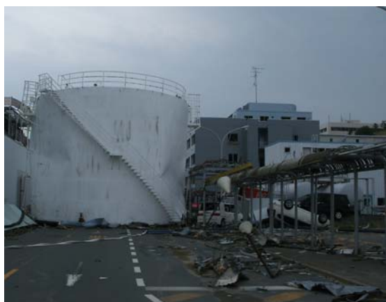
A heavy oil tank washed away in the tsunami onto the road (Diameter: 11.7m×Height: 9.2m)
