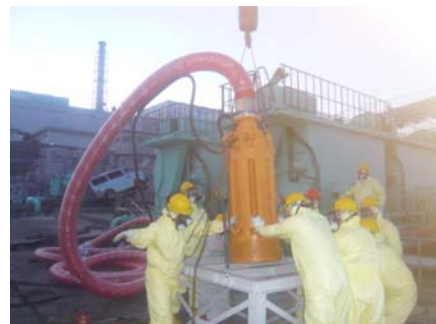
Work conditions for installation of underwater pump
