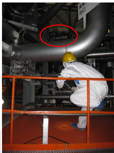
Image of the S/C vent valve inspection work
