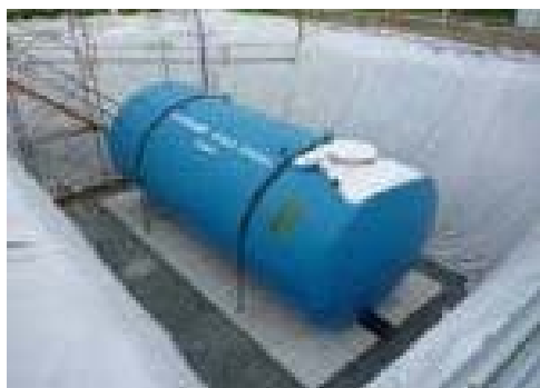
A fire protection tank just before installation
