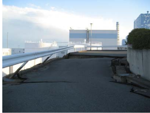
In-site road with cracks that bars vehicle traffic
