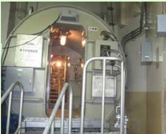
1. PCV entrance (Airlock for workers) (Photo taken on April 17, 2012)
