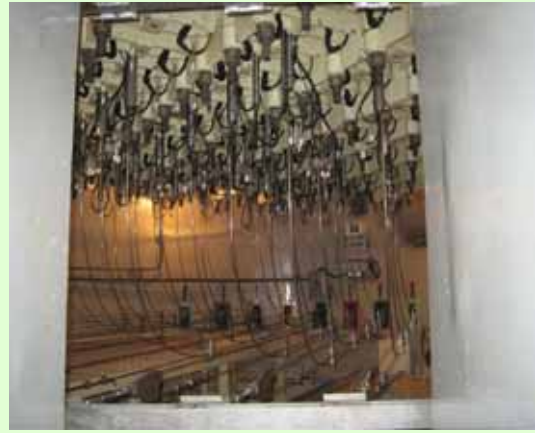
4. Pedestal (Base structure of RPV) (Photo taken on April 17, 2012)
