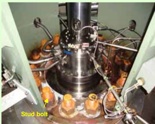
8. Rusted stud bolt on the reactor recirculation pump (B) (Photo taken on February 16, 2012)
