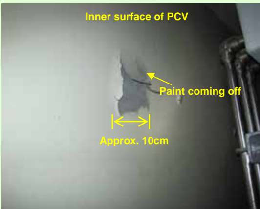
7. Paint coming off on PCV inner surface (Photo taken on March 28, 2012)
