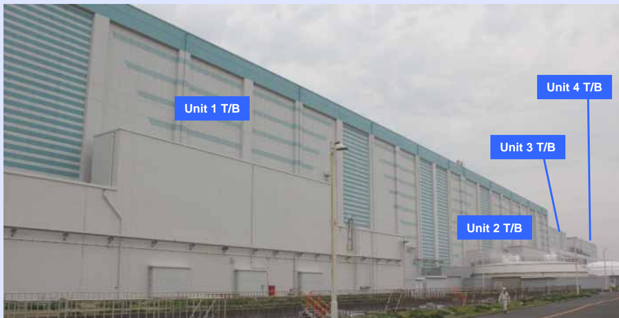
Appearance of Turbine Buildings (Photo taken on May 25, 2012)
