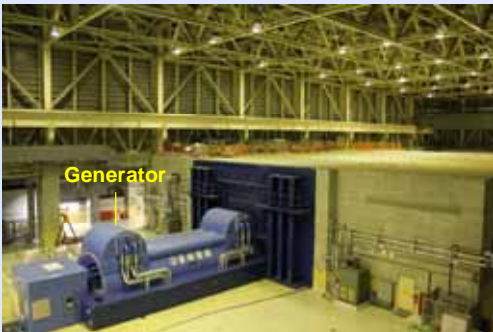
The 2nd floor of Unit 3 T/B (Photo taken on May 15, 2012)
