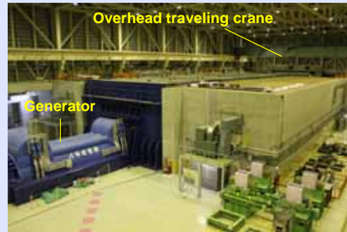
The 2nd floor of Unit 4 T/B (Photo taken on May 15, 2012)
