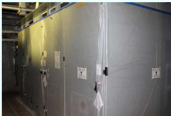
High voltage panel installation completed on November 9, 2012 (Photo taken on December 4, 2012)
