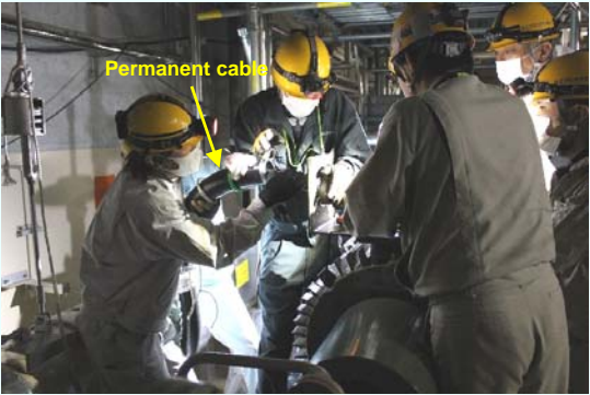
Permanent cable installation (Photo taken on November 21, 2012)
