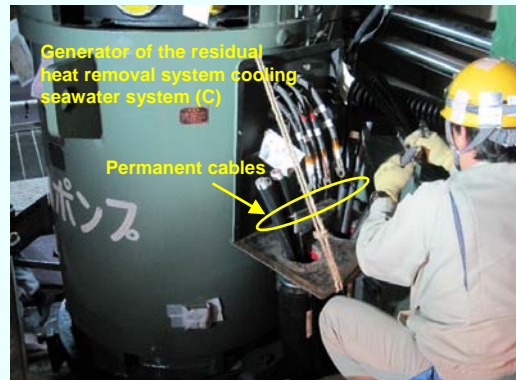
Taking cable core out of the permanent cable for the generator of the residual heat removal system cooling seawater system pump (C) (Photo taken on September 22, 2012)
