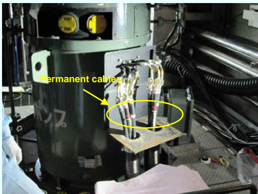
Switching to the permanent cable completed for the generator of the residual heat removal system cooling seawater system pump (C) (Photo taken on November 22, 2012)
