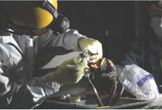
Taking cable core out of the permanent cable (Photo taken on November 21, 2012)
