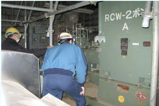
Trial operation [Permanent installation completed on November 29, 2012] (Photo taken on November 29, 2012)
