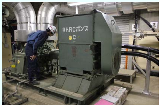
Trial operation [Permanent operation completed on November 28, 2012] (Photo taken on November 28, 2012)
