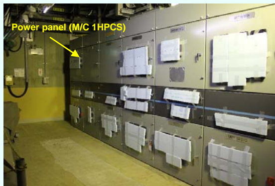
Power panel (M/C 1HPCS) installation completed on November 1, 2012 (Photo taken on November 5, 2012)
