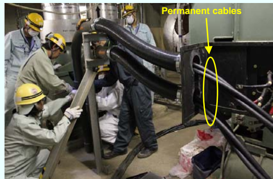
Permanent cable installation (Photo taken on November 20, 2012)
