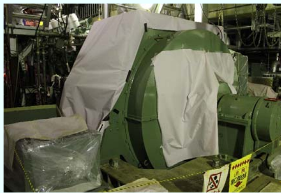
Generator installation completed on November 1, 2012 (Photo taken on November 27, 2012)
