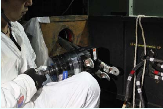
Permanent cable terminal installation (Photo taken on November 27, 2012)
