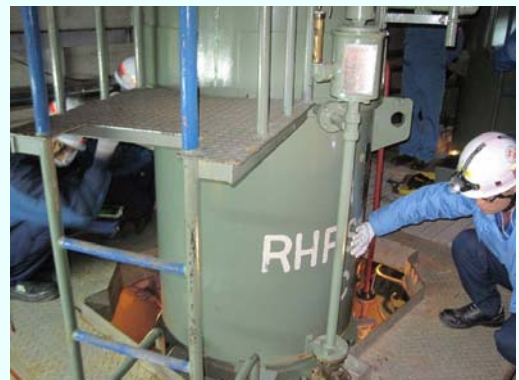
Trial operation of the generator of the residual heat removal system cooling seawater system pump (C) [Permanent installation completed on November 29, 2012] (Photo taken on November 22, 2012)
