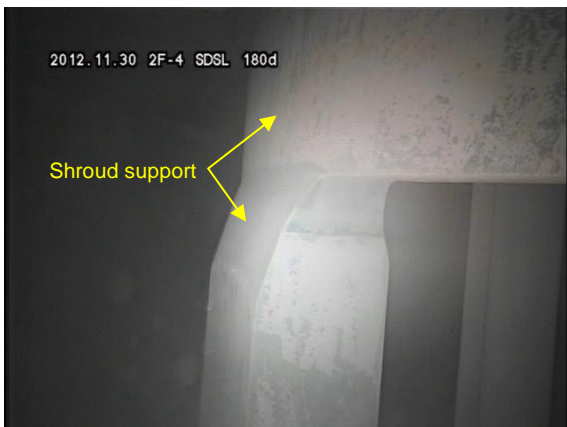
Shroud support (Photo taken in the reactor on November 30, 2012)
