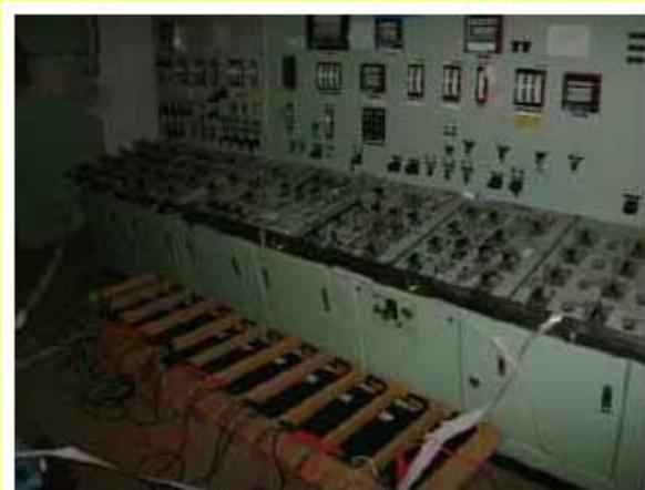
Temporary batteries were used as the power source for measuring instruments
