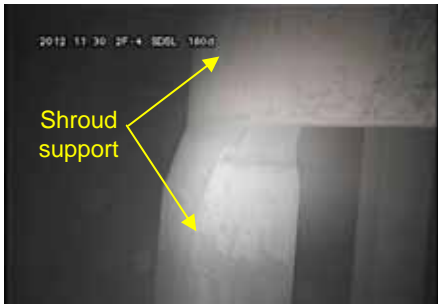
Photo taken in the reactor (November 30, 2012)
