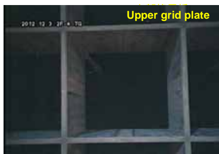
Photo taken in the reactor (December 3, 2012)
