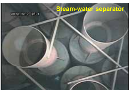
Photo taken in the temporary storage pit for the steam dryer and steam-water separator (December 7, 2012)
