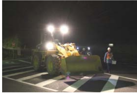
Wheel loader used to secure a route
