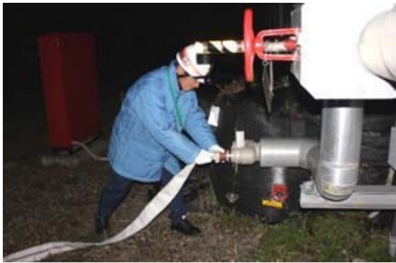
Connecting fire hose to intake on reactor building
