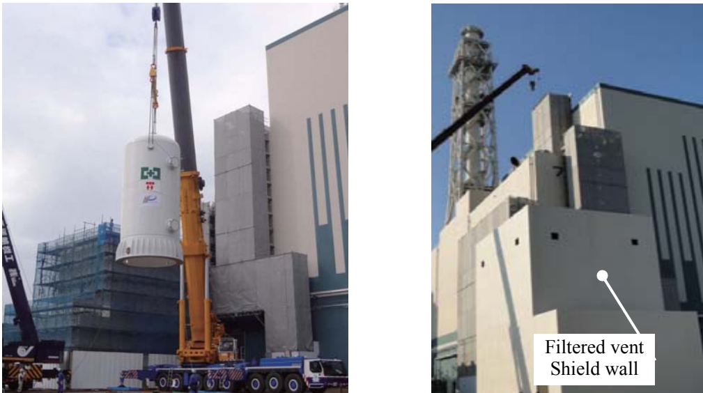
Installing above-ground filtered venting equipment
