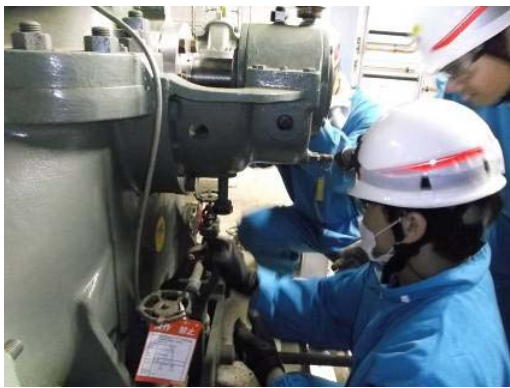
Disassembly (removing attached pipes)
