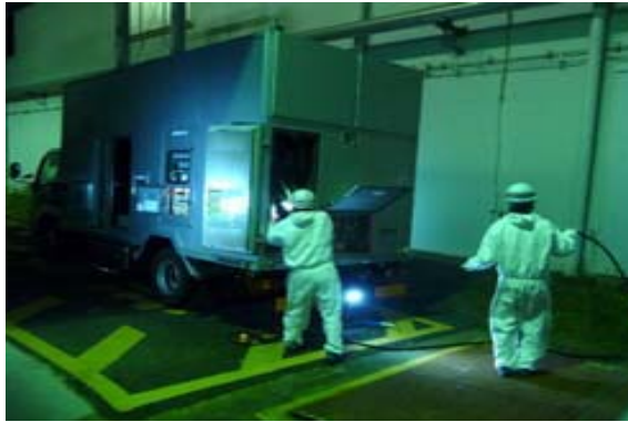
Pulling out cable from power supply car
