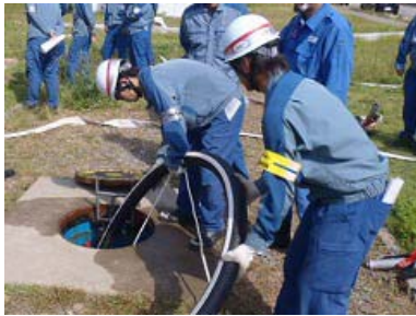
Inserting a suction pipe
