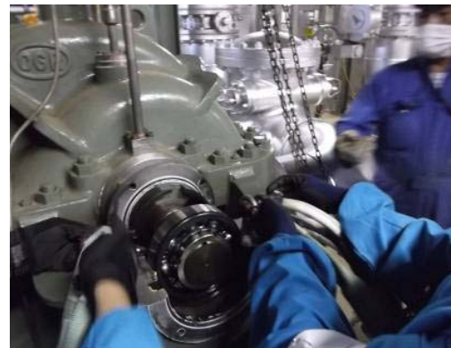
Disassembly (removing bearing cover and case)
