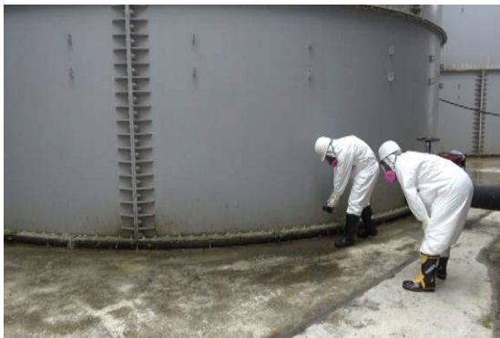
Tank patrol (Geiger counter is used to check for minute leaks from flanges)
