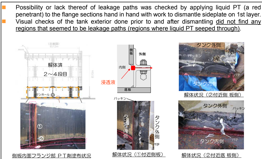
Fig. 2 Investigation Results (1) (results of visual check of sideplate flange surfaces)
