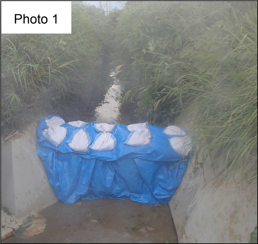
Sandbag dike inside the drainage ditch (8/27)
