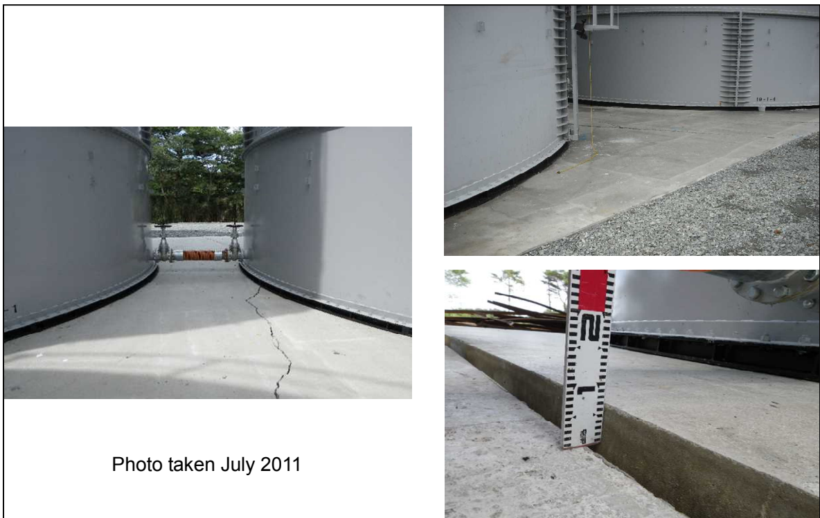
Fig. 2 Condition of the foundation in area H1 east
