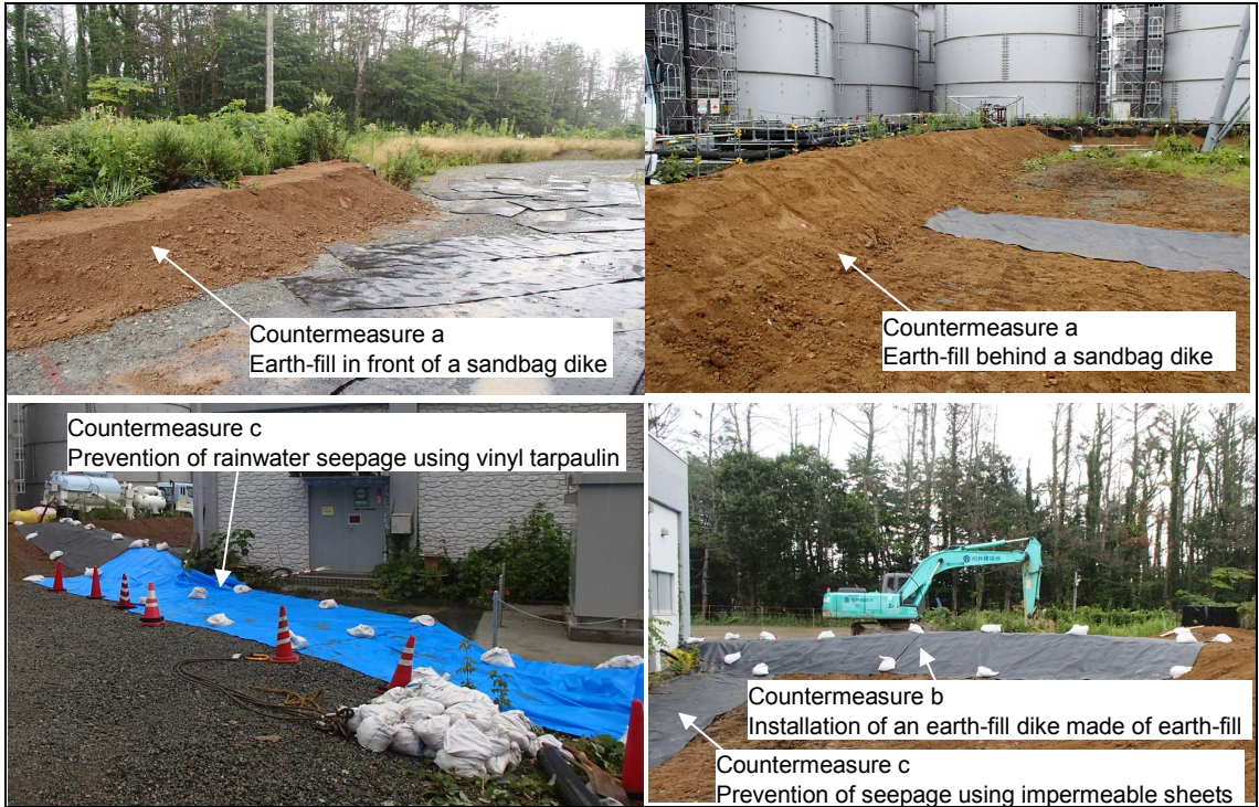
Fig. 4 Installation of sandbags
