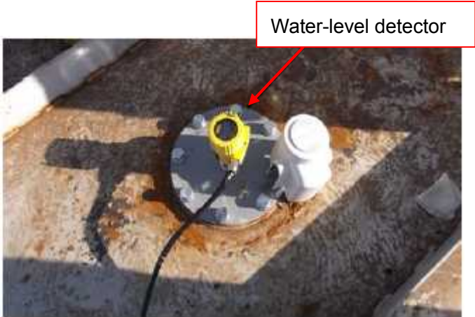
Photo 8 Water gauge installation
