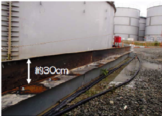
Photo 3 Status of building floodgate embankments using steel plates (area H4 north)
