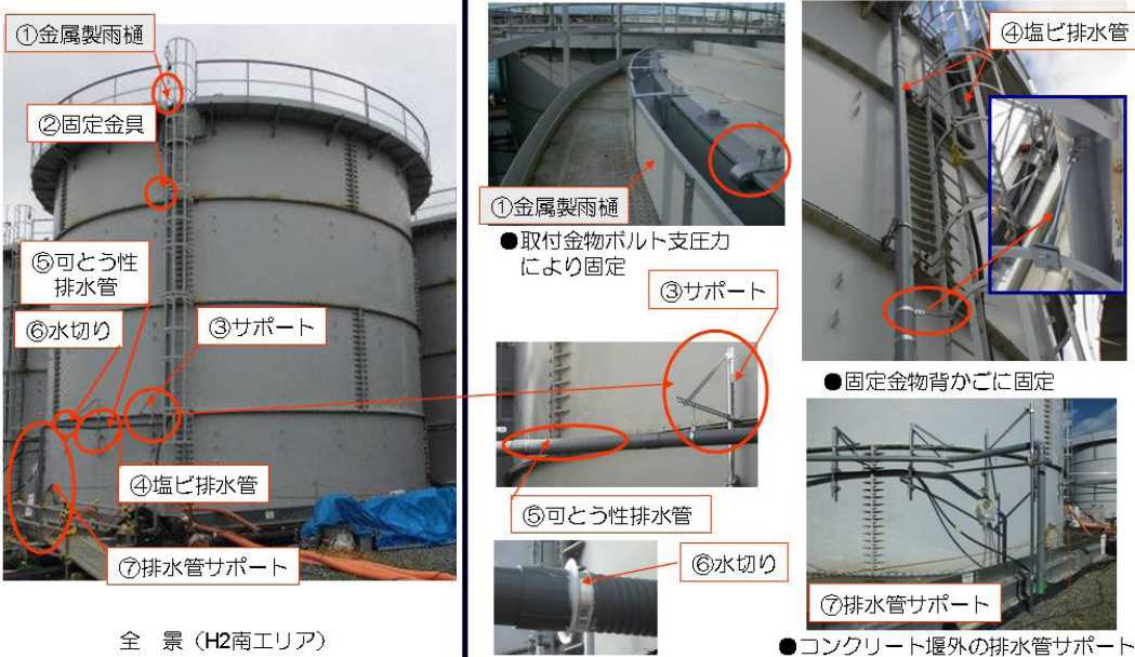
Photo 7 Installation of rain gutters to tank top plate
