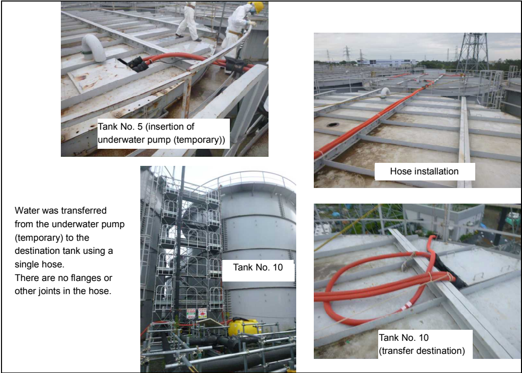
Fig. 2 Installation of underwater pump (temporary) and hose
