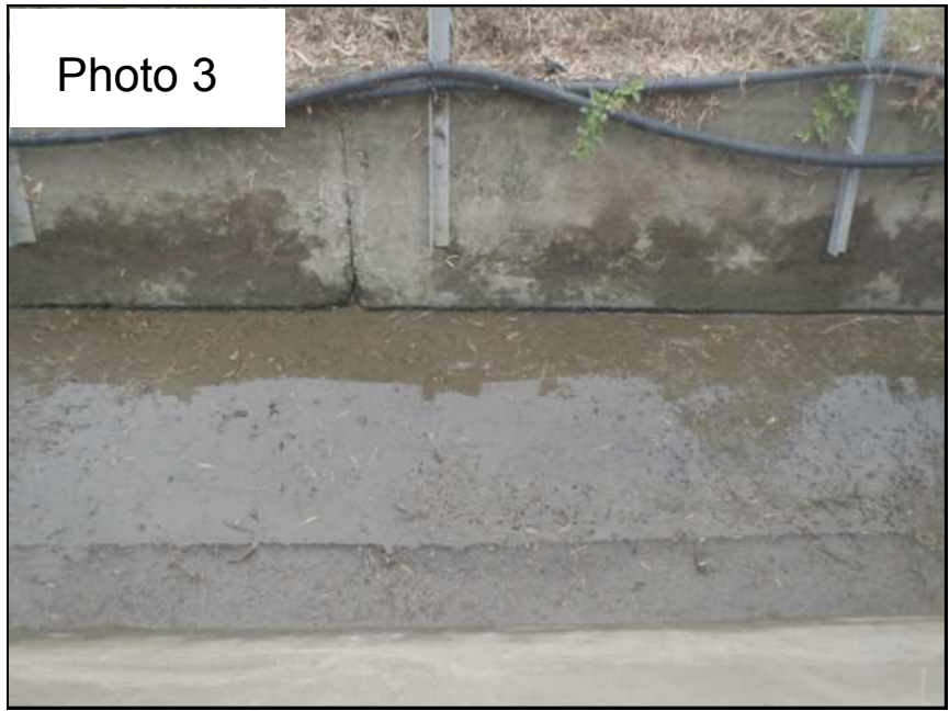
Collection of soil in the drainage ditch (photo taken 9/7)
