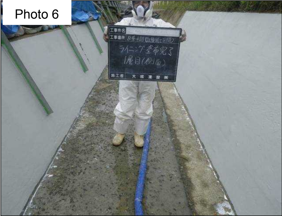
Installation of lining material (photo taken 10/10)
