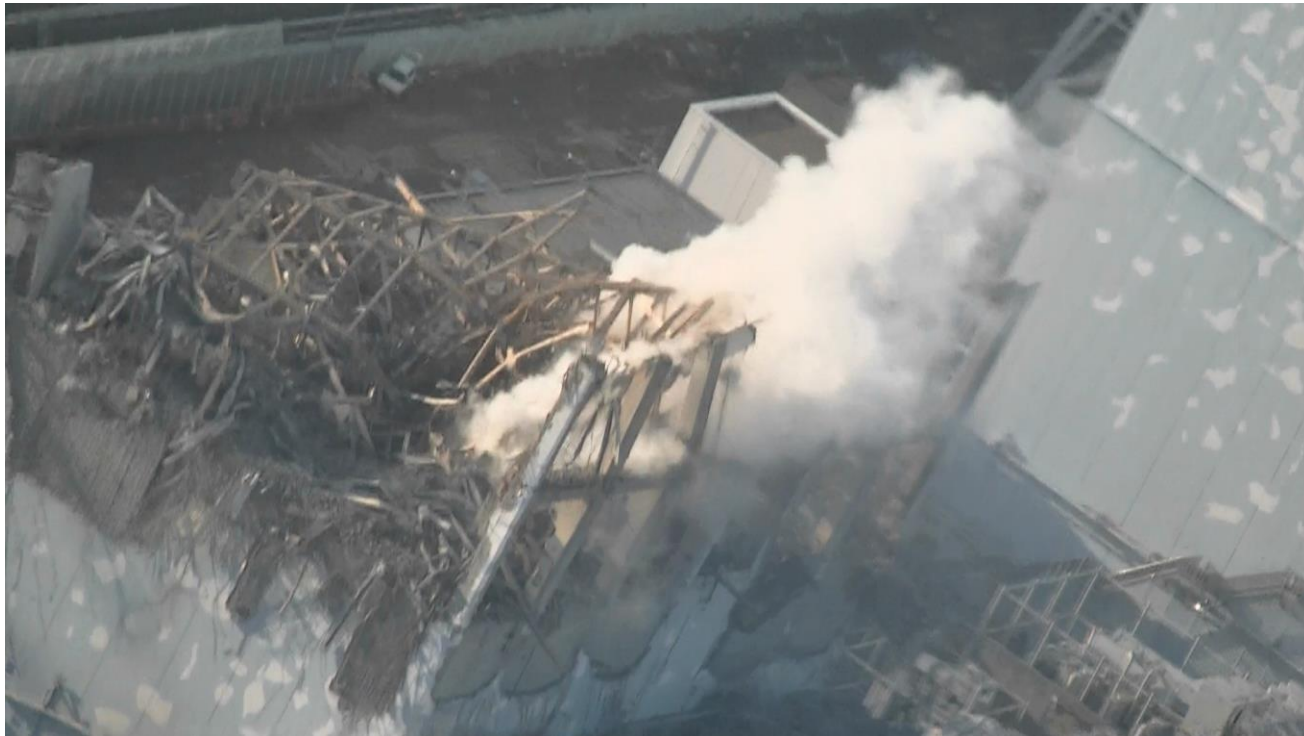
Aerial photo of Unit 3 (March 16, 2011)
