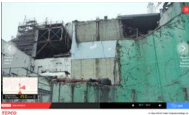
Unit 3 reactor building where a hydrogen explosion occurred
