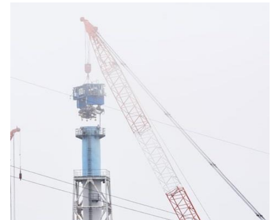
Confirming that equipment can be installed on the top of the exhaust stack
