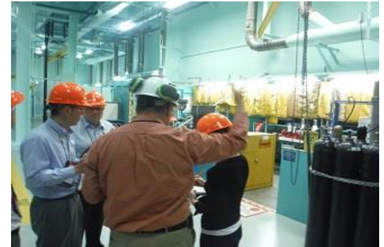
Visit to the Monticello Nuclear Generating Plant (reactor building)
