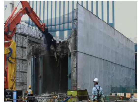
Dismantling of the large freight entrance
