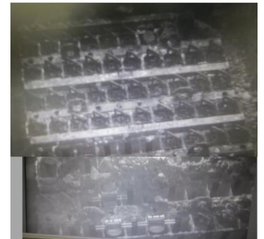
Spent fuel pool after rubble removal
