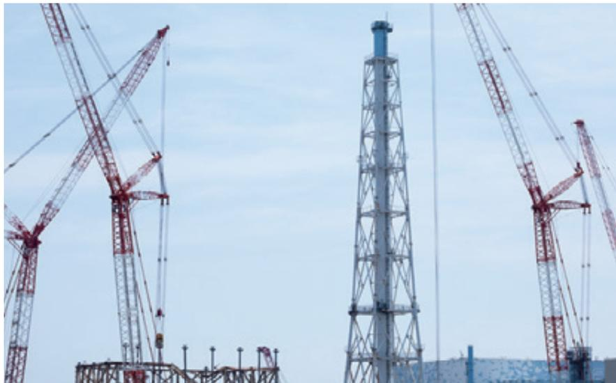
Commencement of dismantling of approximately half of the Unit 1/2 exhaust stack so as to widen seismic-resistance margins (August 2019)
