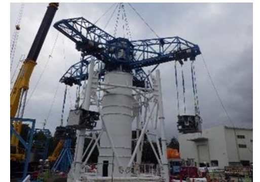
Exhaust stack mockup used for procedure verification
