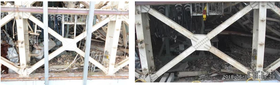
Removal of surrounding steel trusses (left: before removal, right: after removal)
