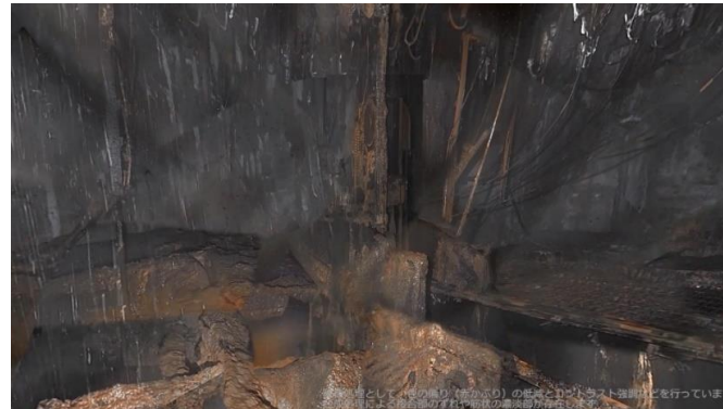
Results of exploration above the platform inside the pedestal
