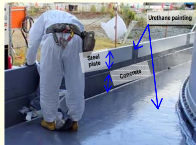
<Status of height increase using steel plates>
