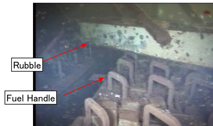
② Rubble and Upper Part of Spent Fuels
