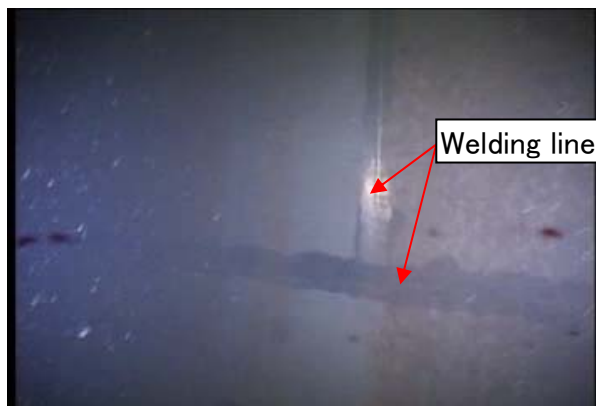
① Southern Wall Surface
